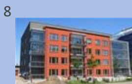
Kv Ishalkan, 201 st, 2013
