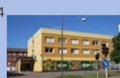
4 Brf Hagahus, 53 st, 2013
