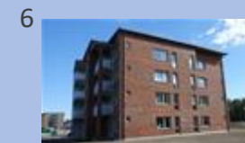
Pyslingen kv3, 324 st, 2016
