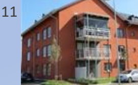
11 Kv Kulan, 174 st, 2011
