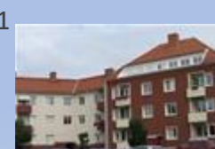
11 Kv Haren, 496 st, 2010
