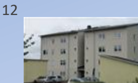
12 Kv Aspsoppen, 190 st, 2002
