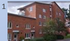
1 Brf Stören, 473 st, 2018
