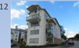
12 Kv Galeasen, 292 st, 2010
